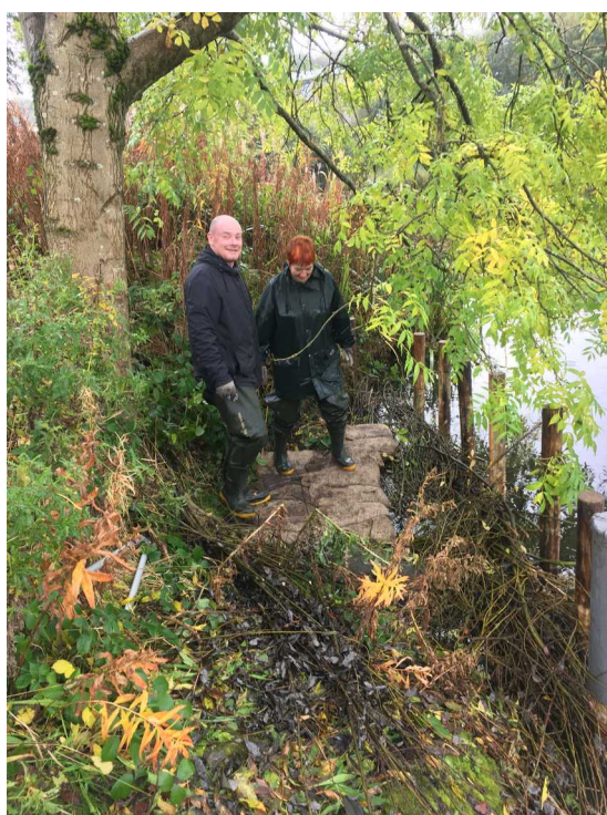
Volunteers from the Ribble Rivers Trust working to improve banks using cut willow bundles from the Wetlands. Stakes are knocked into the water (right of photo), the willow bundles are placed in the water between the stakes and the bank and then hessian sacks filled with soil are placed on top (photo courtesy of the Ribble Rivers Trust).
