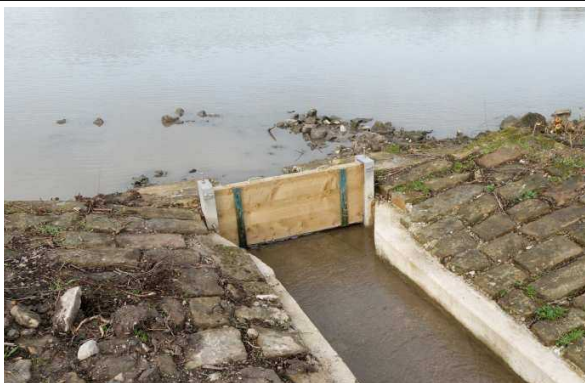
The completed drop-board sluice.
