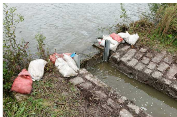
Construction of the sluice – in progress.
