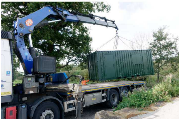
Installation of the storage container.
