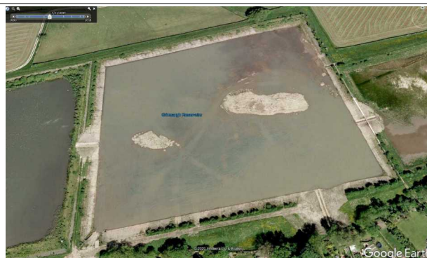
Historical Google Earth image (from 2009) of the central reservoir ('The Island Lake' as it is known today). The, then, newly formed breaches in the embankments and the spillway are clearly visible.
